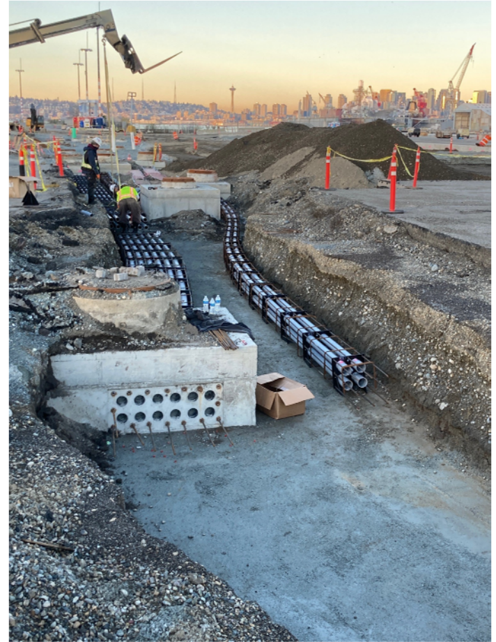
Secondary ductbank at substation
